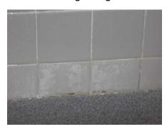
in a piecemeal fashion over the past couple of years. Unfortunately the problem is only apparent when the water begins to permeate the surface and begin to leak through the walls. The appropriate solution for this is to ground out the existing grout and regrout it with an epoxy-based
