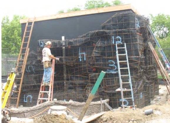
The bobcat holding building was covered with a wire frame which fit together like a jigsaw puzzle to support the rockwork that would cover it.
