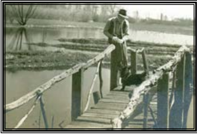
Bridge on 15, Circa 1940
