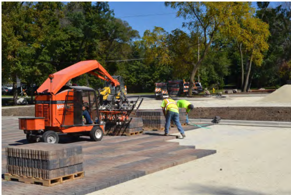
Cosley Zoo leads by example by replacing our parking lot with environmentally friendly permeable pavers.
