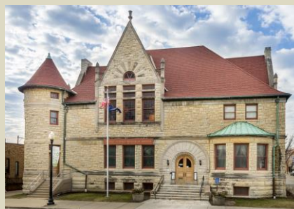
New Museum roof completed April 2016. Photo credit: Larry Kmiecik.
