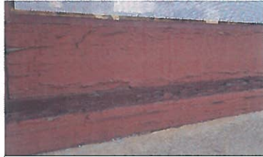
Peeling window frame. Frames up on the west side are worse.
