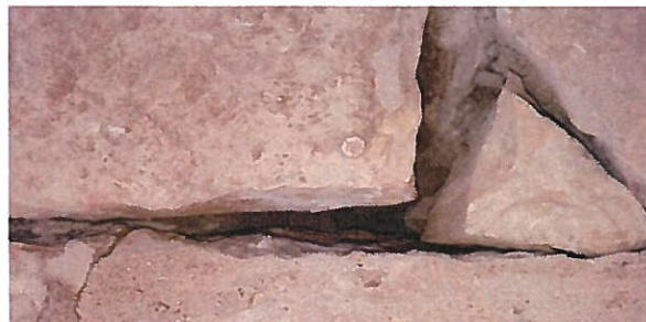
FIGURE A: Cracks and poor adhesion between the mortar and the masonry units within the body of the obelisk are clearly visible once exterior stones are removed. The stone unit at bottom right has detached from the mortar and is in danger of falling from the monument. During the mortar removal process we found stones units not attached to the backup.
