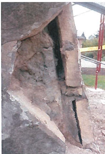
FIGURE A: Cracks and poor adhesion between the mortar and the masonry units within the body of the obelisk are clearly visible once exterior stones are removed. The stone unit at bottom right has detached from the mortar and is in danger of falling from the monument. During the mortar removal process we found stones units not attached to the backup.
