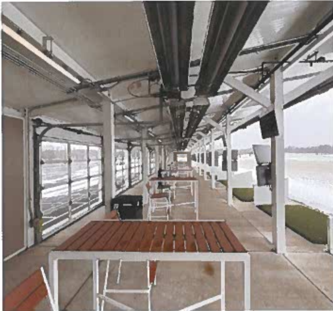
Base Bid Radiant Tube Heaters
