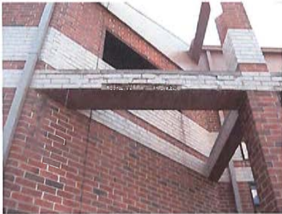
Faces of bricks at courtyard area have popped loose from the structure due to freeze-thaw cycles and moisture infiltration.
