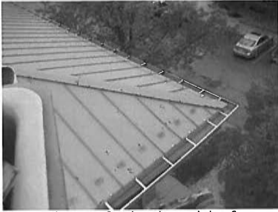
Another area of moderately corroded roofing.
