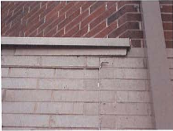
Metal coping cap over existing stone coping at entrance canopy. Note narrow vertical control joint with sealant squeezed out of joint.
