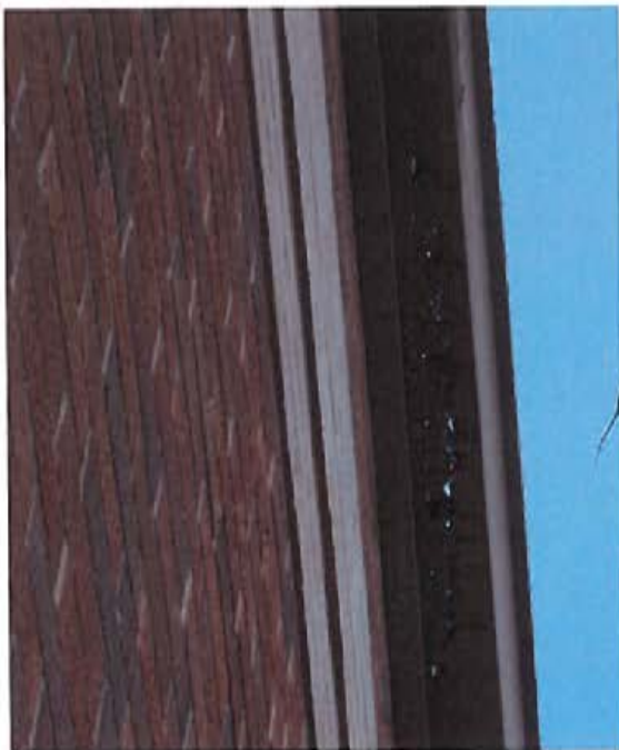
Some sections of original gutters are completely corroded through and no longer perform as intended.
