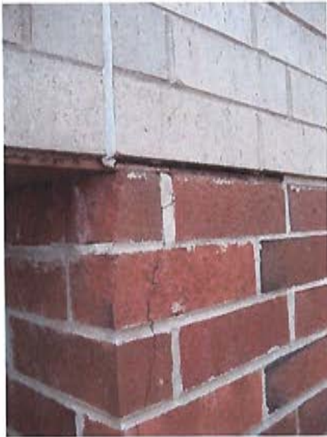
Minor cracking at lintel conditions.
