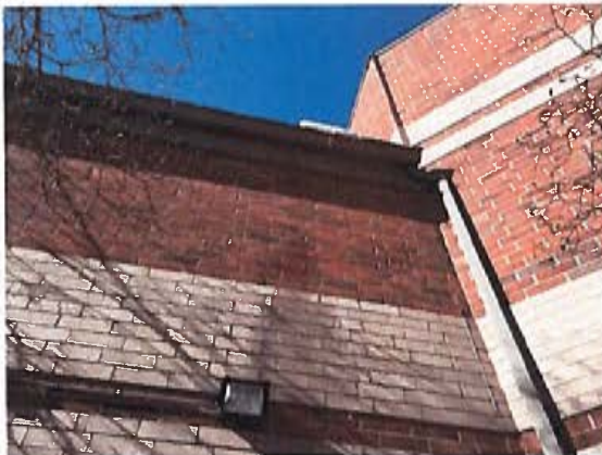
Gutter and downspout damage is evident at several locations.
