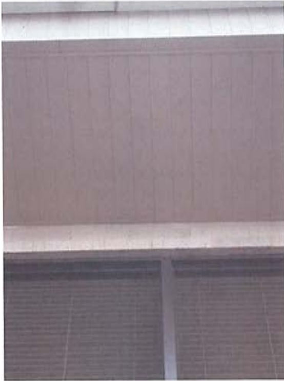
Metal soffit and fascia panels are generally in good condition throughout the facility.
