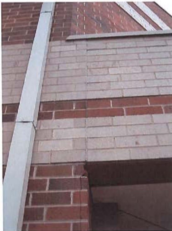
End of existing entrance canopy. The small vertical control joint at the end of the canopy is of insufficient size to accommodate thermal stresses, resulting in damage to the brick masonry below.
