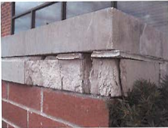
Deteriorated masonry at partial-height wall cap
