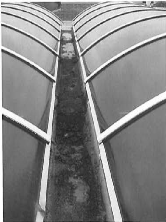
Modified bitumen roofing between skylights above the lobby has minimal slope and should be actively monitored for water intrusion.
