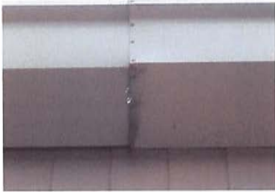
Corrosion and popped rivets at gutter seams are creating leaks at several locations.
