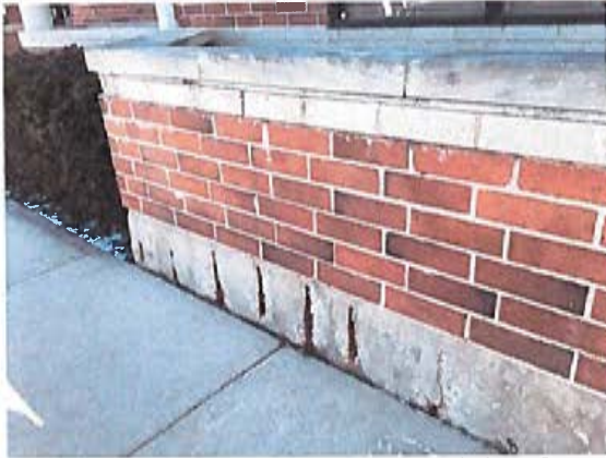
Masonry deterioration and exposed, corroded reinforcing steel at concrete wall base
