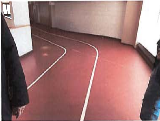
Banked corners at tracks are showing moderate to severe wear and are in violation of ADAAG guidelines for cross slope.
