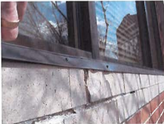
Aluminum flashings installed at window sills allow for wind-driven moisture to enter the wall assembly underneath the flashing piece.
