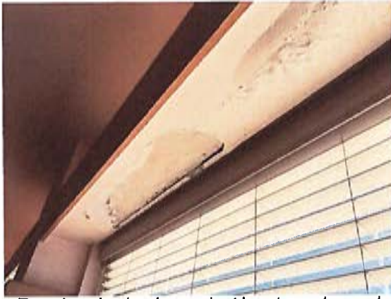
Typical window head at track with moisture-damaged drywall.
