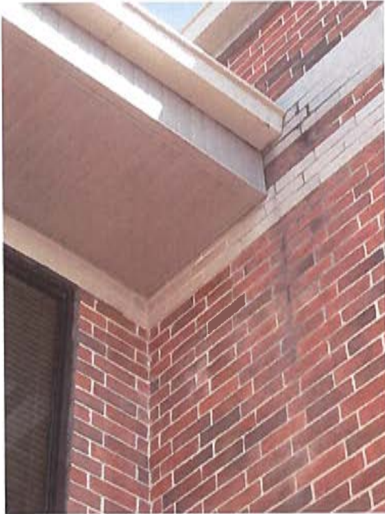
Another example of water staining at gutter ends. The use of diverter strips on the roof above will divert concentrated amounts of rainwater from ends of gutters. This location is an example of where an additional downspout would improve performance.
