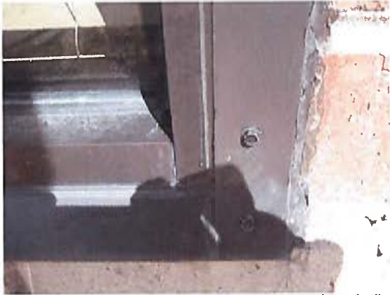
Sealant repairs and additional flashing at jamb and sill conditions. Sealant in this location is beginning to deteriorate.
