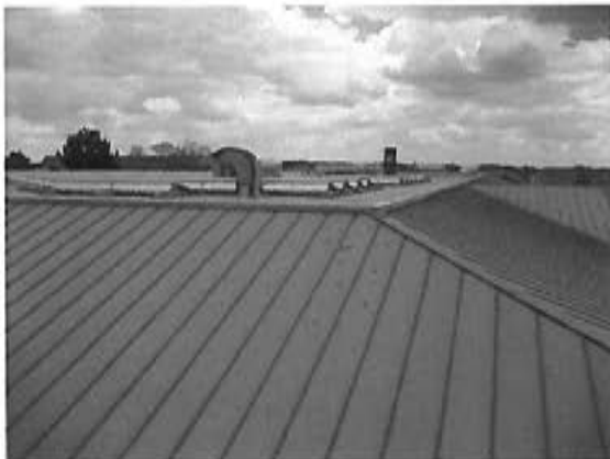
Most of the standing seam metal roofing on the facility has experienced deterioration of finish, and corrosion is becoming more and more visible with time.
