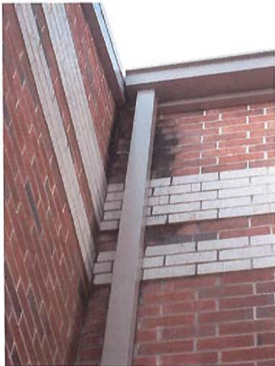
Example of masonry staining behind downspouts.
