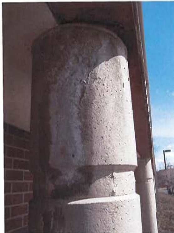
Freeze-thaw deterioration at top of existing stone column covers. Note sealant repairs and corroded steel lintel at top of column.
