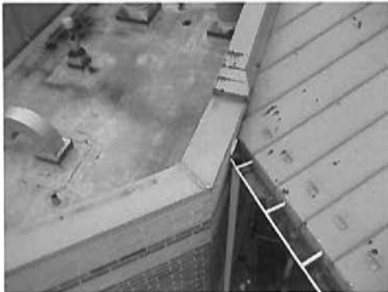
Example of corrosion at standing seam metal roofing and metal copings.
