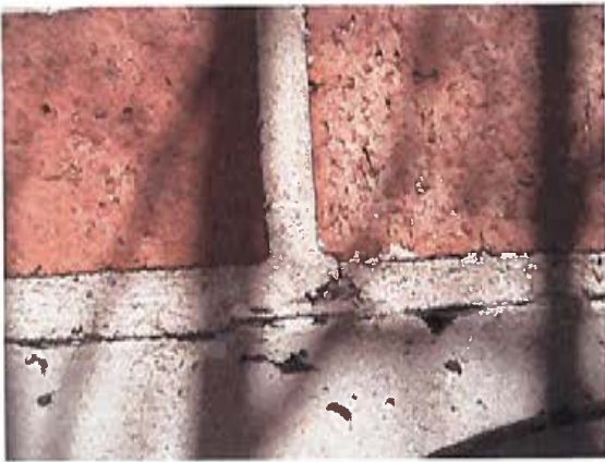
Typical sash cord weep at base of wall assembly is severely deteriorated.
