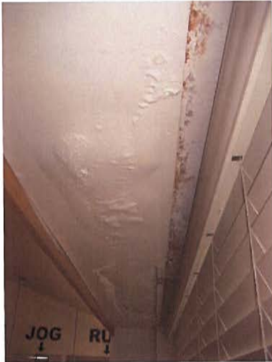
Close-up photo indicates drywall construction in contact with steel lintel.
