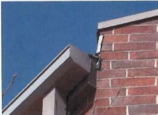
Example of gutter end where repairs have been made to prevent water intrusion and masonry damage.
