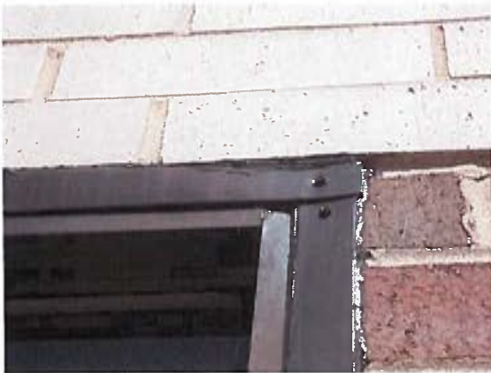
Head and jamb flashings. Sealant above head flashing is blocking the flashing and weep path of the wall assembly, inhibiting escape of moisture from the building.
