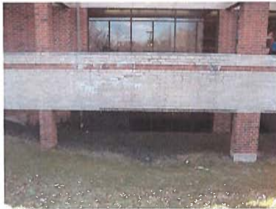
Faces of bricks at courtyard area have popped loose from the structure due to freeze-thaw cycles and moisture infiltration.
