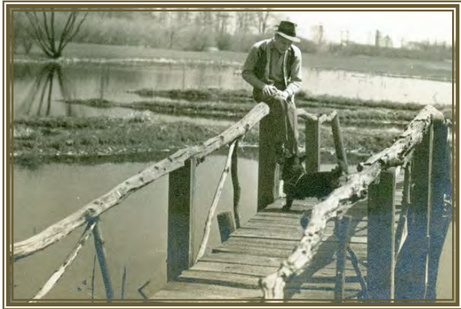
Bridge on 15, Circa 1940
