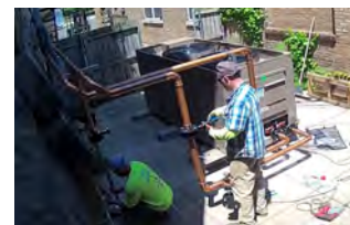
HVAC vendor piping in new chiller. Michelle Podkova
