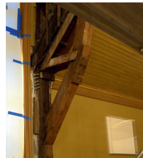
An exposed beam during the construction project. Emily O'Brien
