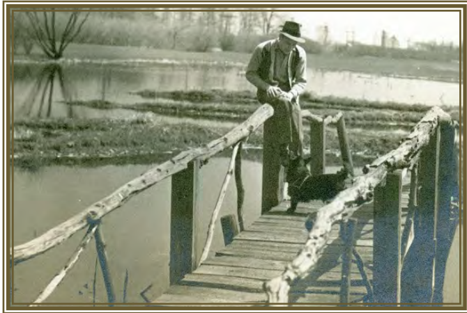
Bridge on 15, Circa 1940
