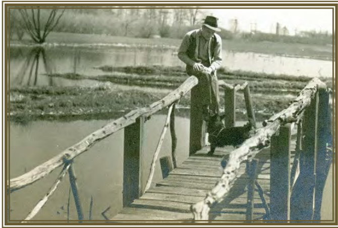
Bridge on 15, Circa 1940
