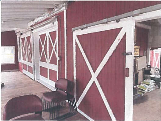
Figure 7. East elevation under the covered patio.
