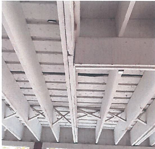
Figure 20. Underside framing of the cover porch
