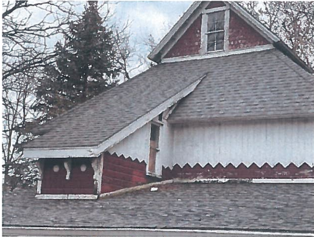
Figure 14. Second story view of the East elevation
