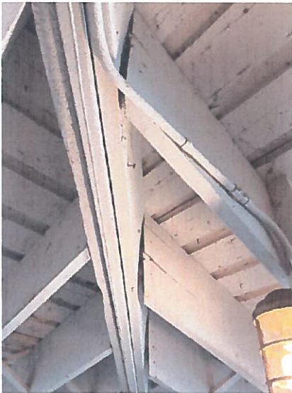
Figure 19. Framing at the underside of the cover porch.
