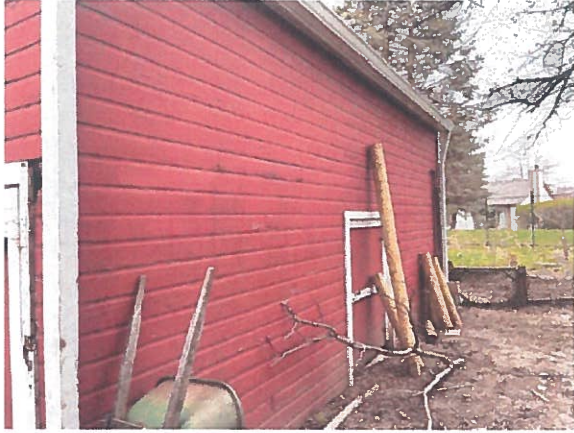
Figure 10. West elevation of the lean-to addition
