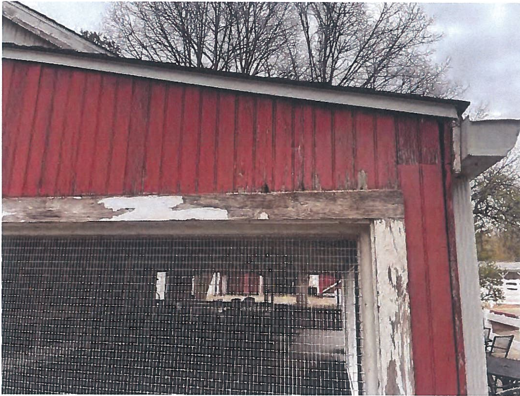
Figure 12. Deterioration at the wood clapboards and frame of the opening at south elevation
