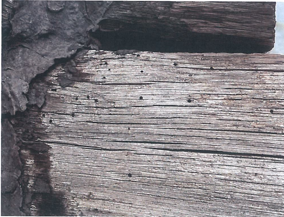
Figure 36. Infestation and woodpecker damage at west elevation
