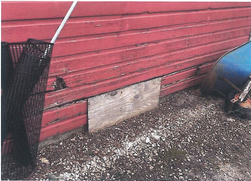
Figure 11. Deteriorated and missing clapboard on the original portion of the barn.
