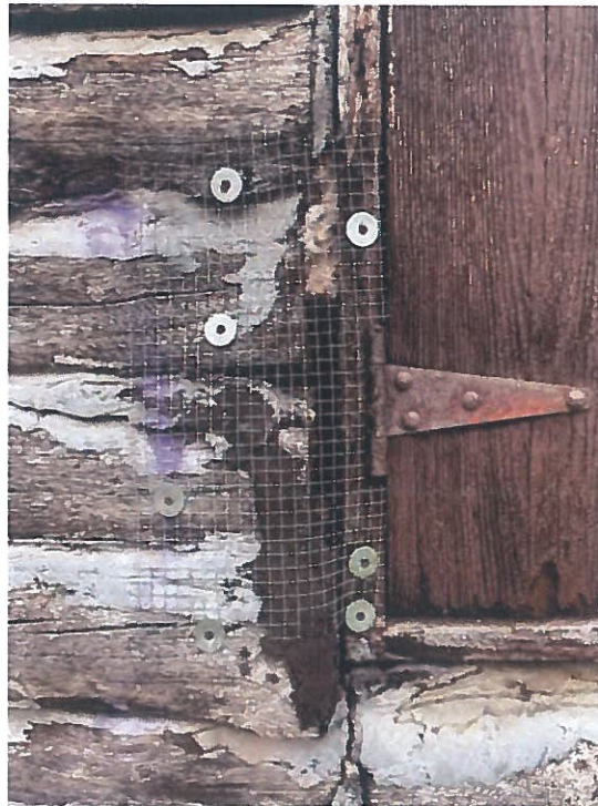
Figure 34. Hole adjacent to Window frame and damaged wood
