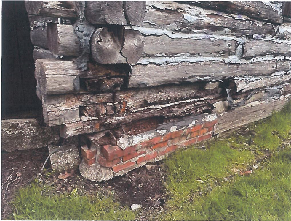
Figure 32. Deterioration of Wood logs at corner notching
