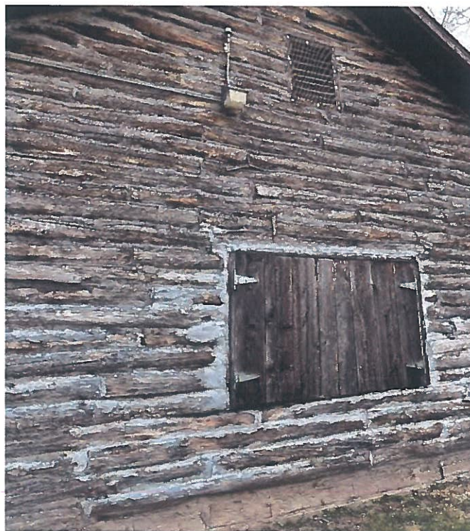
Figure 33. Mastic material at east elevation
