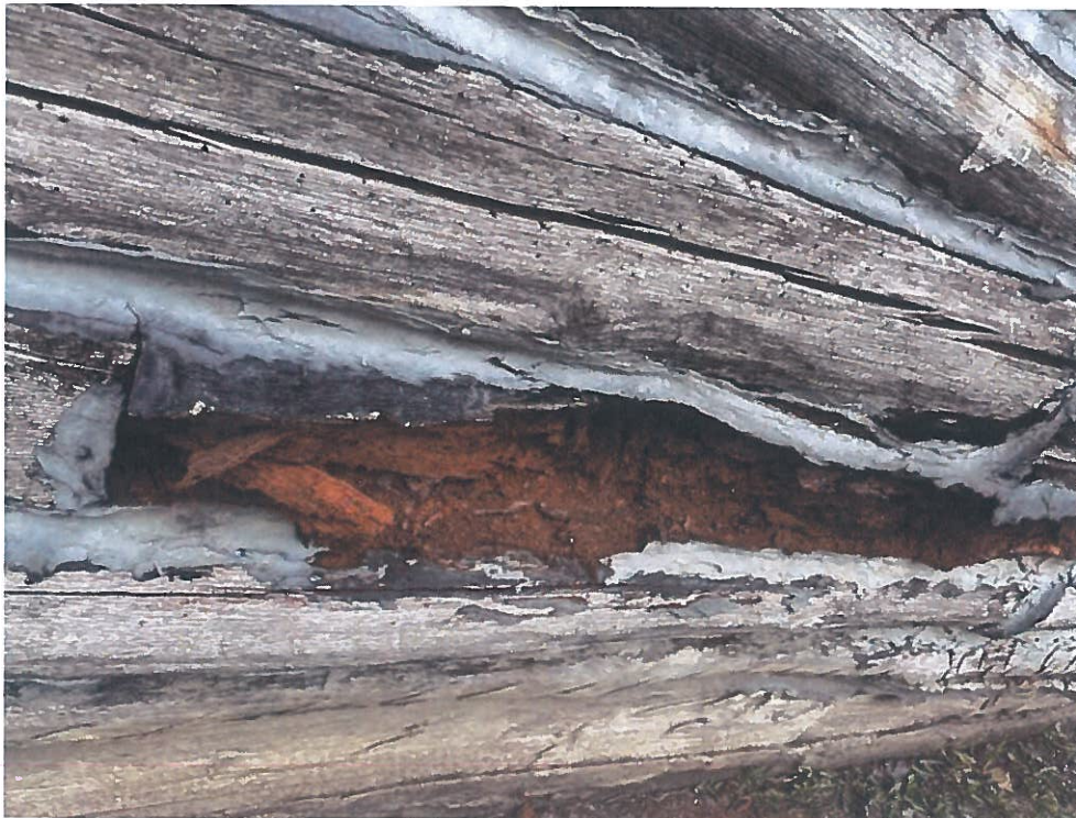
Figure 37. Infestation at west façade
