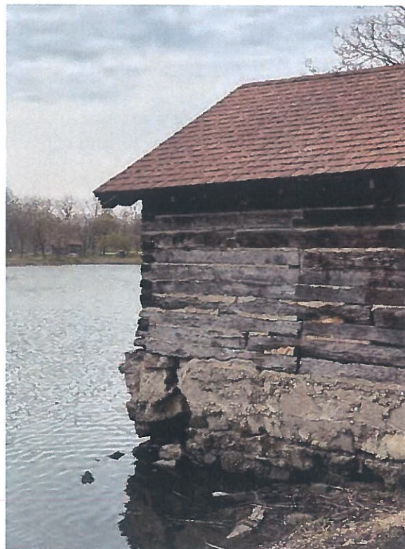
Figure 43. Cracked foundation in critical condition at southwest corner
