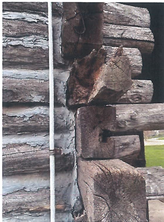
Figure 35. Broken wood log at notching
