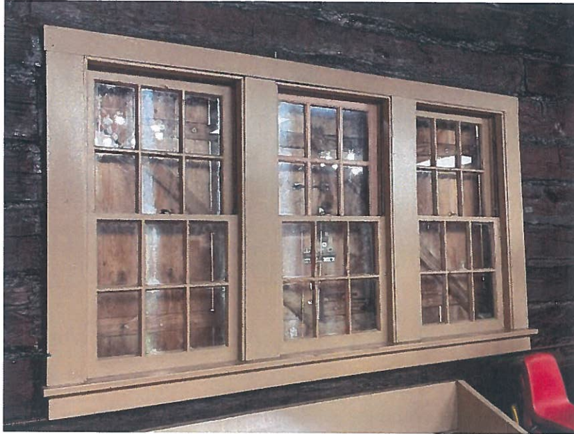
Figure 38. Double-hung windows at the Girl Scout Cabin protected by wood boards from the outside
