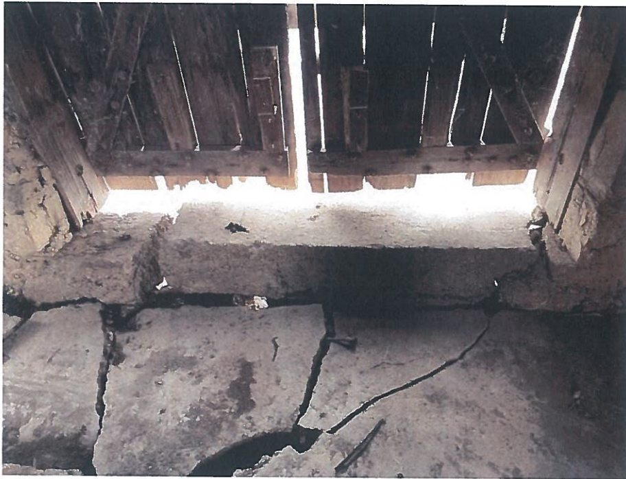
Figure 47. Cracked concrete floor near door on west façade
