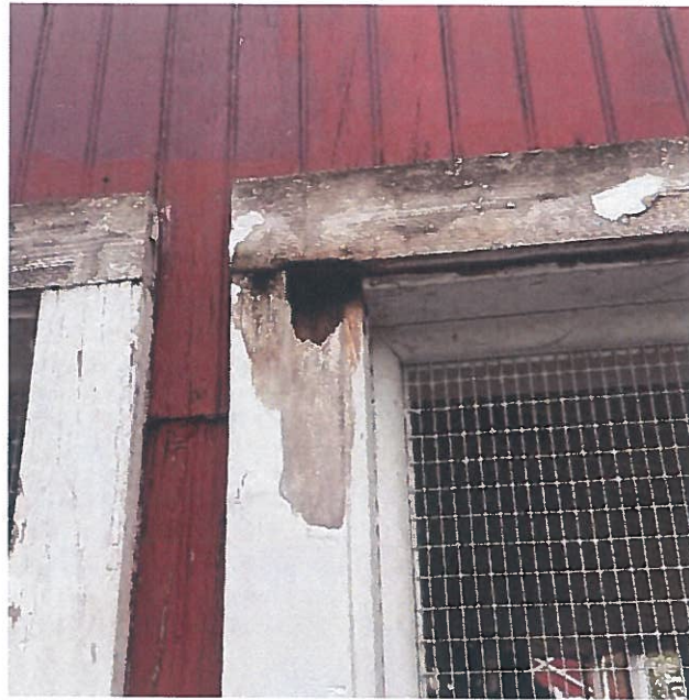
Figure 18. Damage at the frame of the opening
