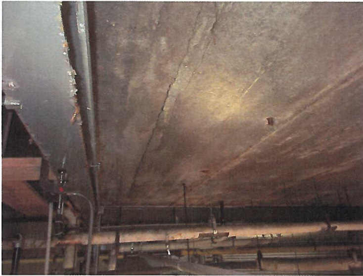
Photo 15: Crack in the hollow core plank at the underside of the 'attic' space
