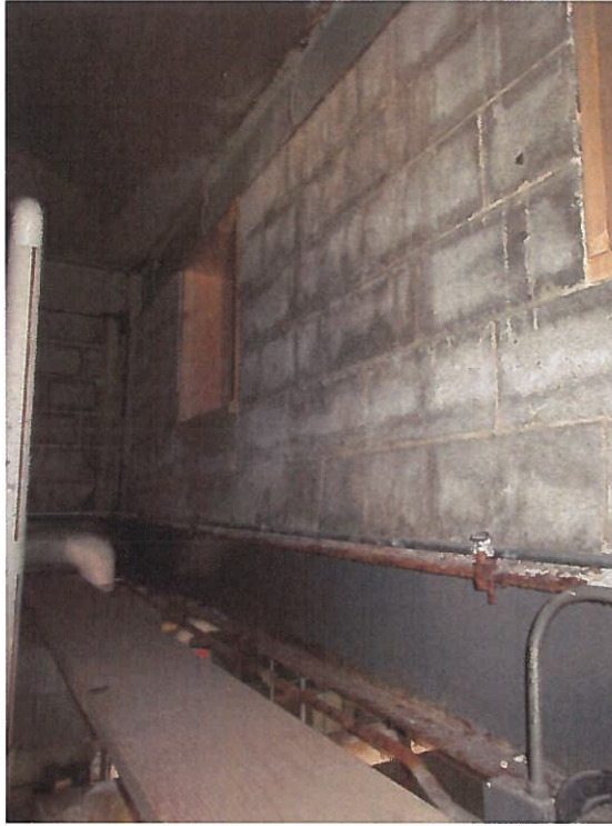
Photo 17: CMU knee wall enclosing 'attic' spaces, note existing steel beam below the wall which also supports the edge of the plank parallel to the span.
