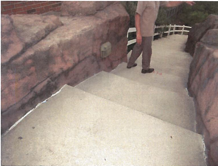
Photo 10: Concrete stairs and sealant joint at base of rock work
