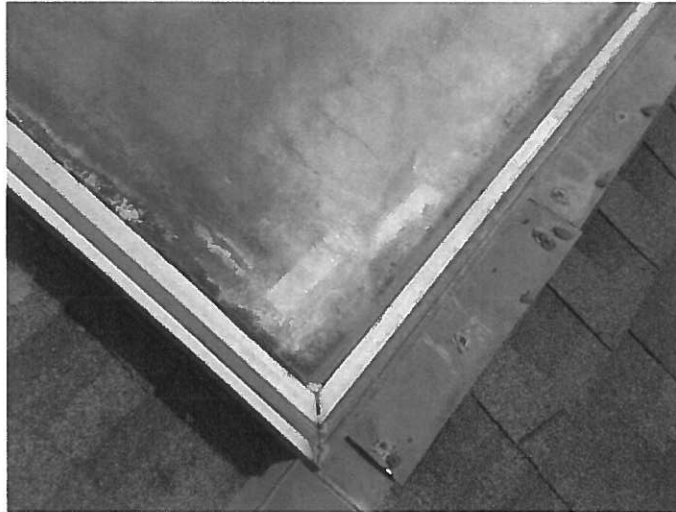
3. LEAKING SKYLIGHT SEAL
