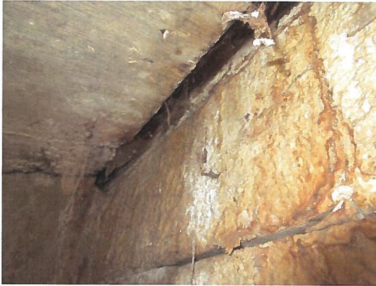
Photo 21: Salt deposits on CMU wall below expansion joint at south end of stair
