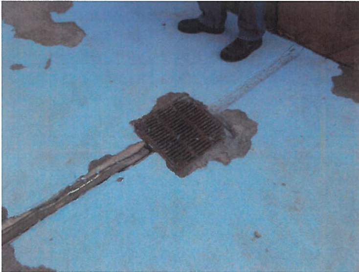
Photo 6: Failed expansion joint at landing, note existing drain location
