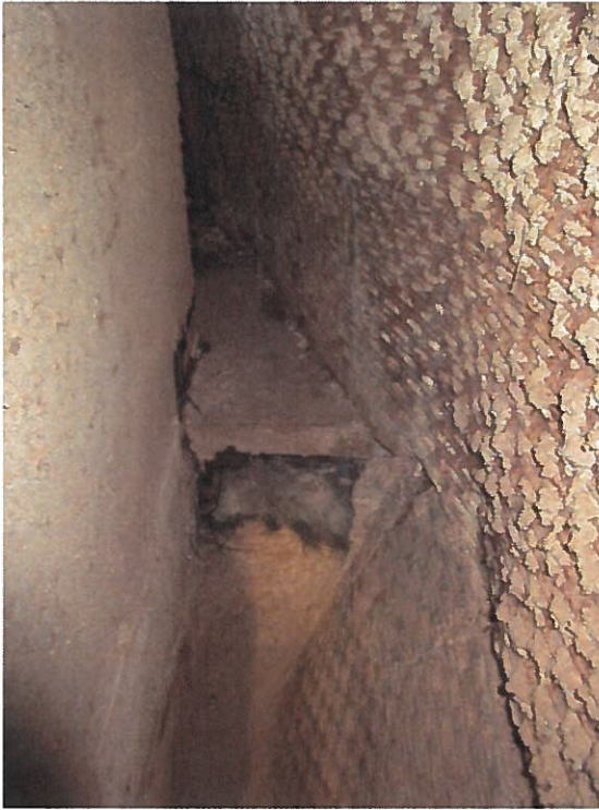
Photo 13: Edge of split slab system at landing access to waterslides, note the black roofing material below the concrete topping
