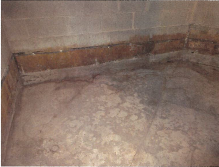
Photo 11: Top of concrete plank at floor of 'attic' space below rock work (after roofing material was removed)
