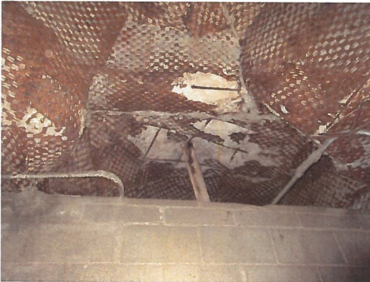
Photo 22: Deteriorated metal lath below rock work
