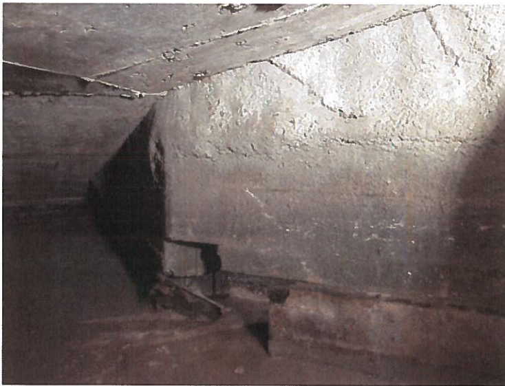
Photo 20: Condition of the CMU walls between the 'attic' spaces, note shotcrete at the top of the walls.
