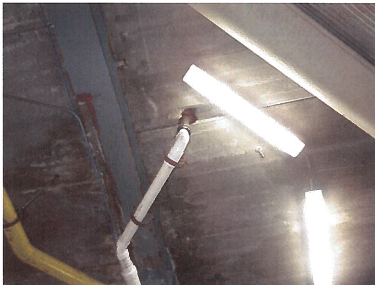
Photo 18: West end of the hollow plank with rust staining
