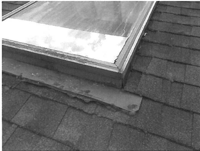
1. DETERIORATED SKYLIGHT
