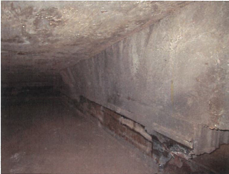
Photo 12: Top of concrete plank at 'attic' space below stairs (after roofing material was removed)
