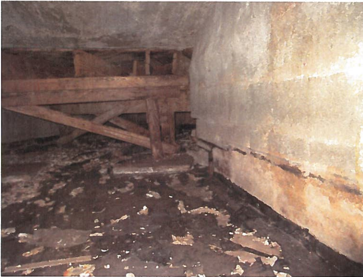
Photo 4: Original roofing membrane at floor of 'attic' space
