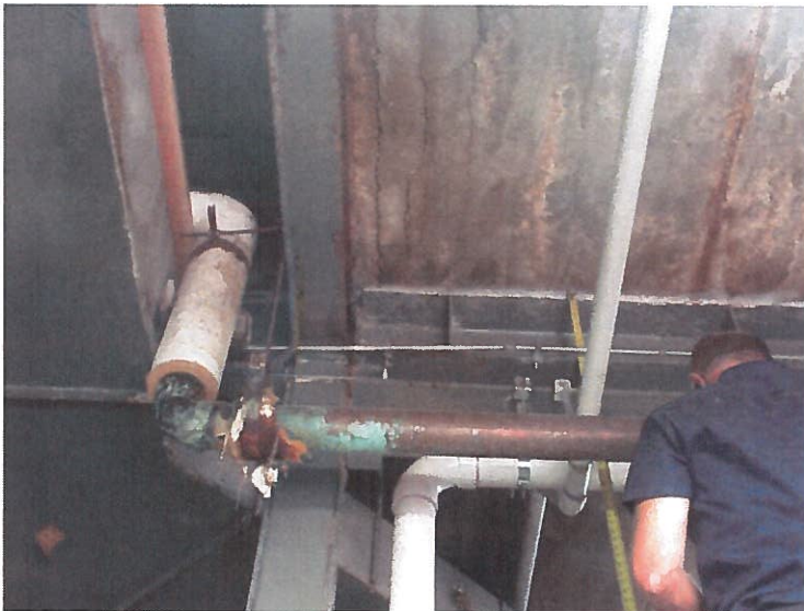
Photo 16: West end of hollow core plank supported on Col. Ln. 1
