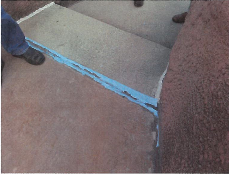
Photo 5: Expansion joint at top of concrete stair and topping of landing to waterslides.
