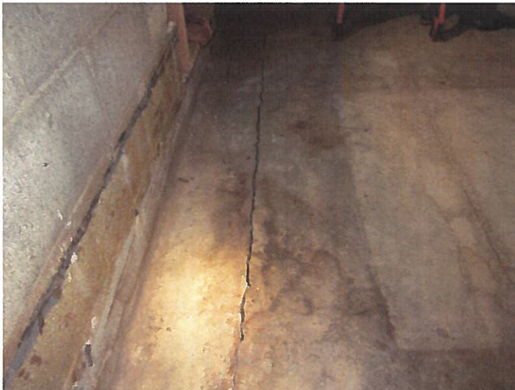
Photo 14: Crack at the topside of the hollow core plank in the 'attic' space.
