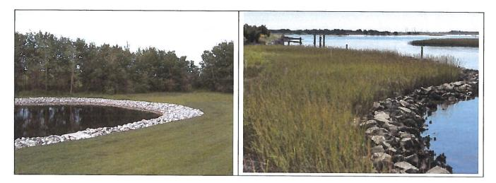
• Provides long term armoring of the side slope which is tolerant to fluctuating water level, however does not allow vegetation to grown along shoreline
