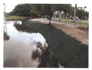
• Provides structural stability to pond side slope during periods of fluctuating water level. Also, allows for "natural" pond edge as plants become established.
