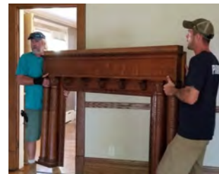
Carpenters move the mantel. Michelle Podkova
