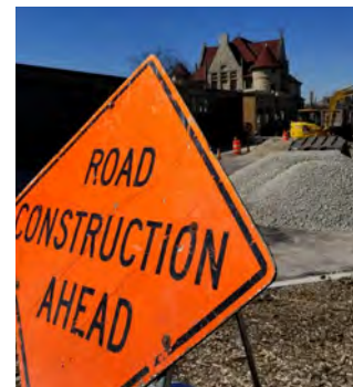
Construction in front of the Museum, Summer 2019.
