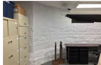
Storage space remediation project results. Photo credit: Morgan Valenzuela
