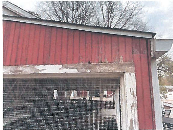
Figure 12. Deterioration at the wood clapboards and frame of the opening at south elevation
