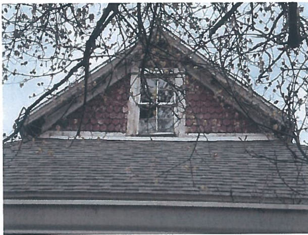
Figure 15. Upper portion of the west elevation. Note broken windowpane.
