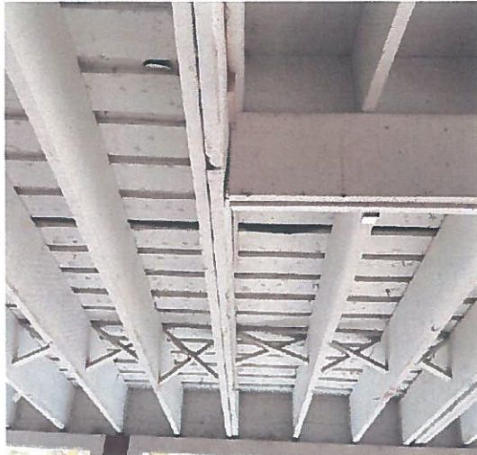
Figure 20. Underside framing at the cover porch
