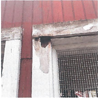
Figure 18. Damage at the frame of the opening
