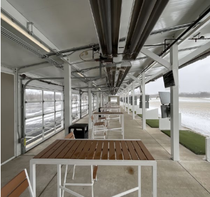
Base Bid Radiant Tube Heaters
