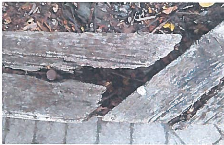
Examples of rotted timbers
