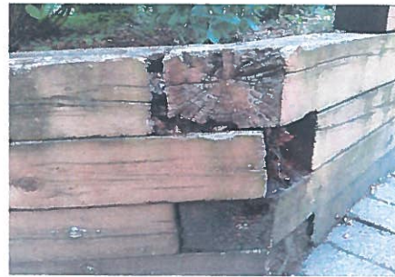
Examples of rotted timbers
