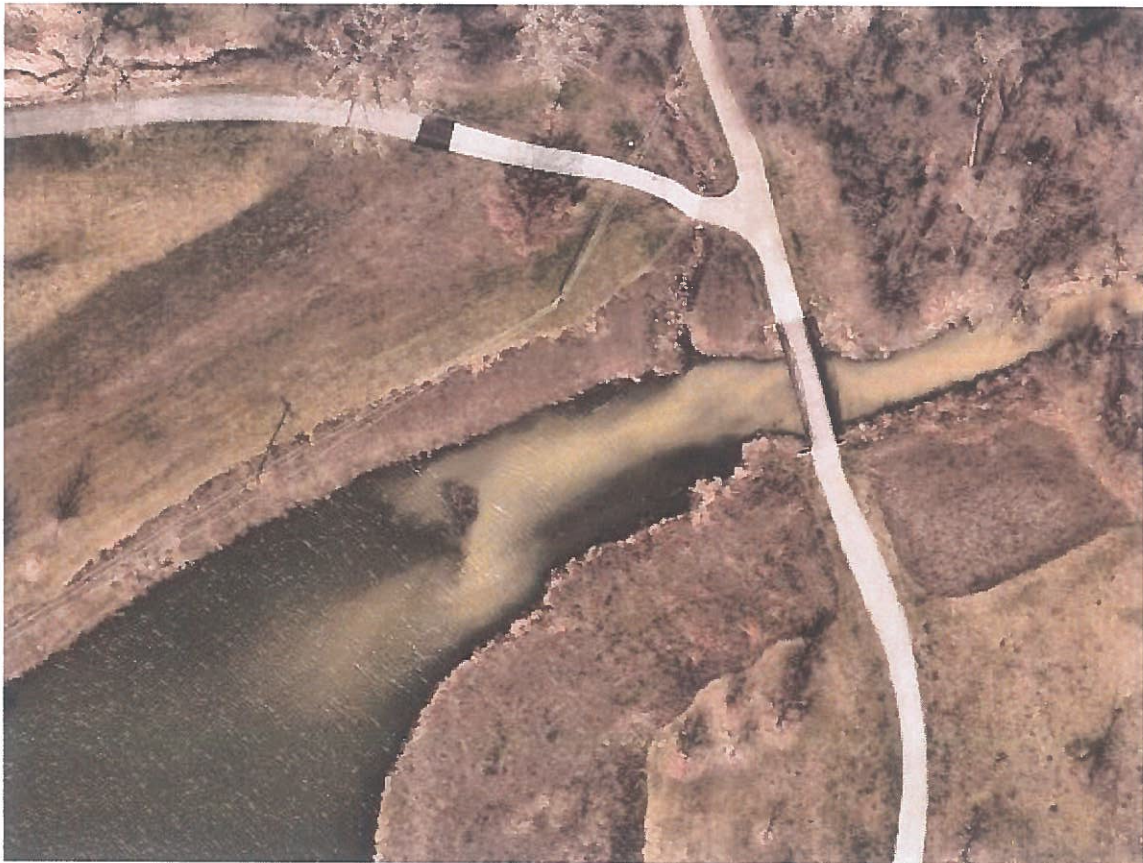
Figure 1 – North End of Sediment with debris/tree blockage (March 2024):
