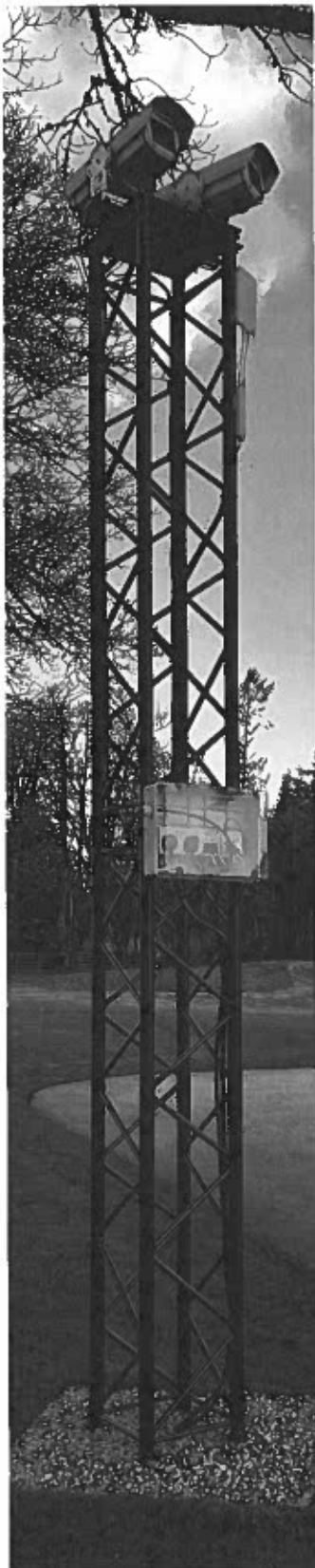
An example of a concrete foundation for a truss holding the sensors.
