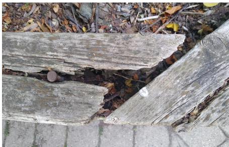
Examples of rotted timbers
