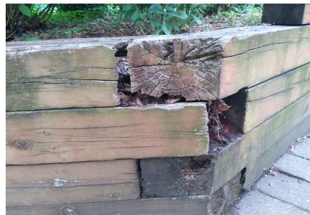
Examples of rotted timbers
